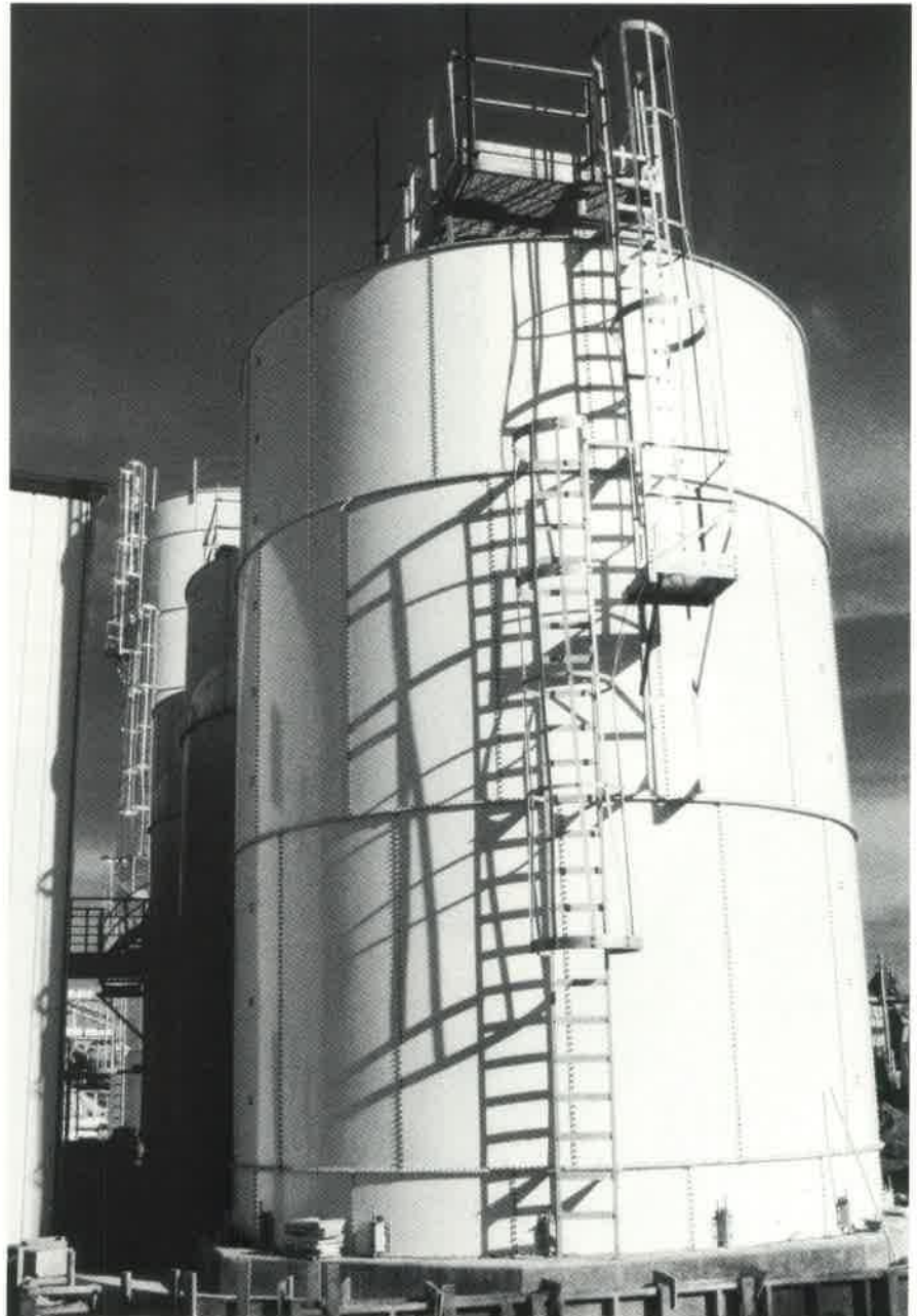
Precipitated calcium carbonate is stored for use by an adjacent paper mill.
